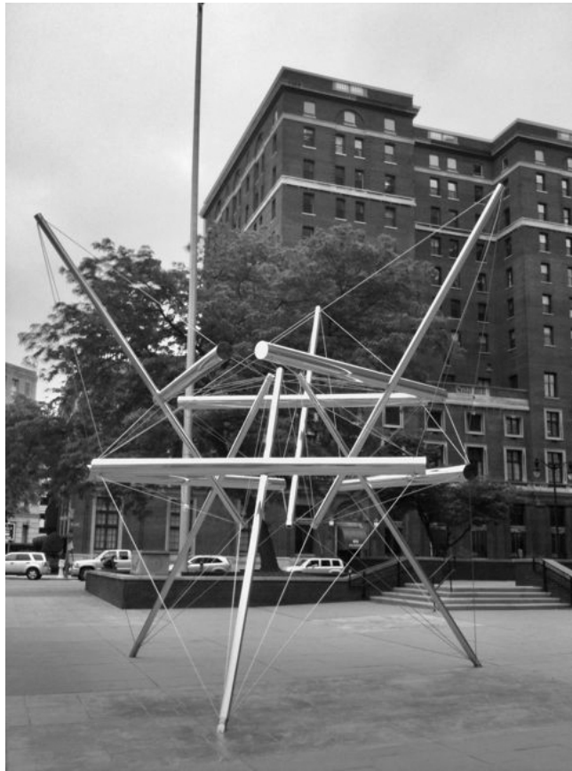
Figure I.8.5 A tensegrity structure on a plaza in Buffalo, NY, USA. The tall vertical that extends to the top of the frame is a flagpole in the background. (Photo by the Author)
